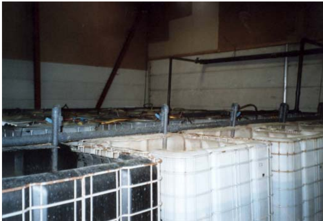
Fig. 11. The recirculation system constructed by Greenfish. The system is placed inside a barn that is usually used for agricultural purposes. The fish is farmed in the containers in the front of the picture. Water is flowing through pipes to the basin. The waste water is then pumped to the biological and mechanical cleaning that is conducted in the containers in the back of the picture. The clean water is then pumped back to the fishes. The system is closed and uses a minimal input of water. (Photo: Berggren, 2007)
